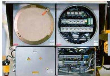
The type of protection of panel boxes for Zone 1, Zone 2 and Zone 21 on crane and hoist combines flameproof enclosure »db«, increased safety »eb« and protection by enclosure »tb«.
