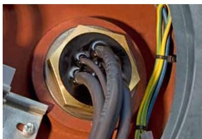
Indirect cable entry, extremely high safety level, provided by protection types increased safety »eb« and flameproof enclosure »db«. Connection from the Ex e connection box to Ex d is by means of post-type bushings.
